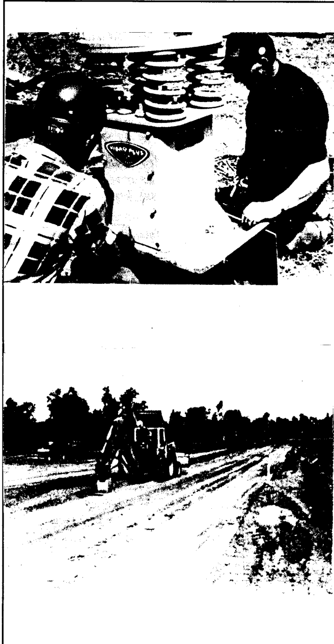
Figure 5-5. Special equipment for compacting sand in pervious toe trenches
